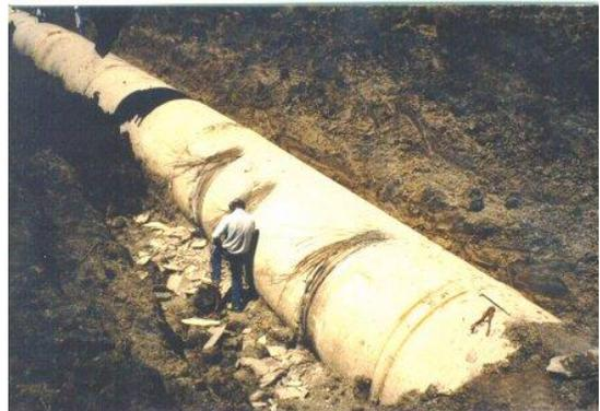
Figure 14. Deterioration detected by monitoring
