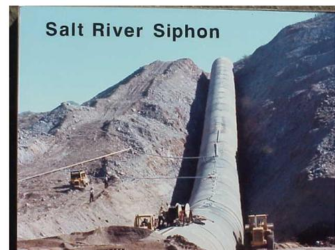
Figure 2. 21-foot diameter PCCP pipeline
