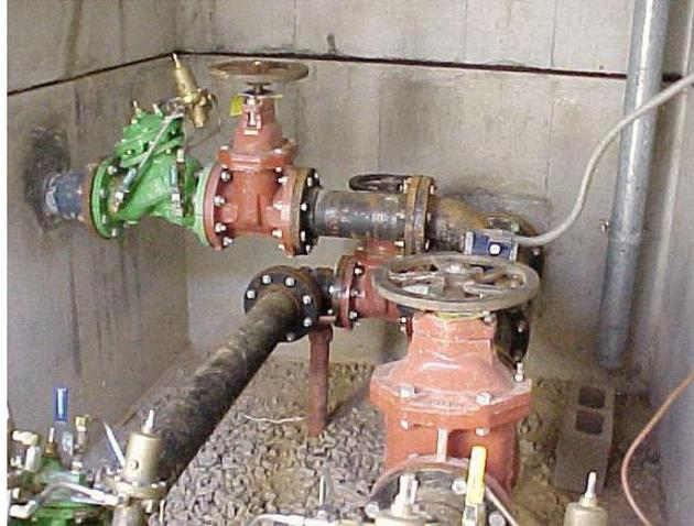
**Figure 3 – Pressure Reduction Valve**
